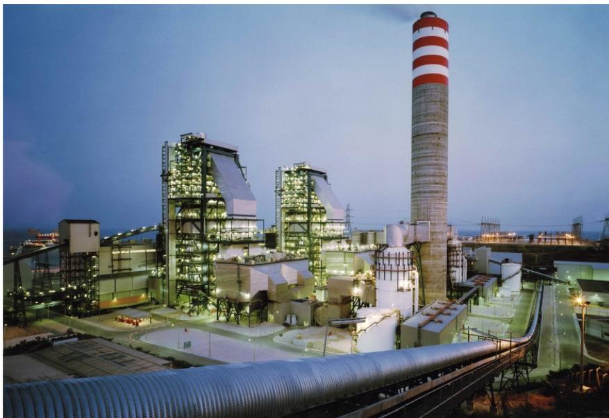
*The 1320 MW Sugozu power plant. The plant consumes up to 30 kt/d of imported hard coal delivered via one of the world's largest floating coal trans-shipment terminals. This handles 3 Mt/y of coal, delivered mainly by Capesize vessels from Colombia and South Africa (photograph courtesy of STEAG)*
