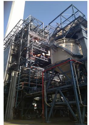
*REACT regenerative coke-based system for multipollutant control at the Isogo Plant in Japan*
