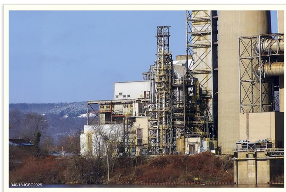
Figure 18 ECO 2 post-combustion 1 MW pilot demonstration at R.E. Burger Plant in Ohio, USA (courtesy of Powerspan)
