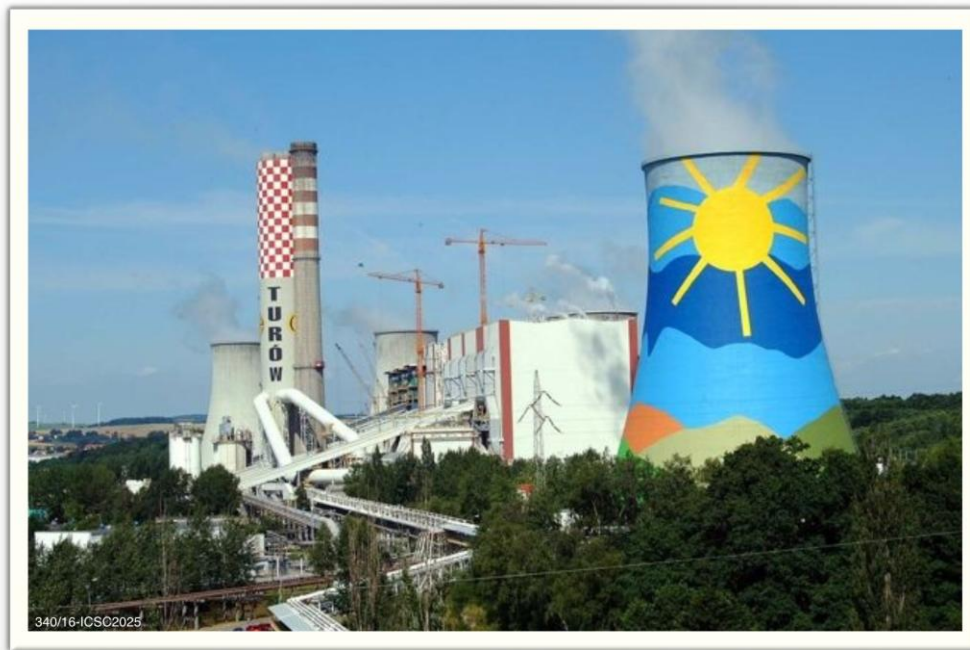
Figure 16 Turów CFBC power plant, Poland (courtesy of PGE)
