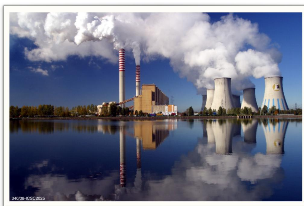
Figure 8 Bełchatów coal-fired power plant, Poland (courtesy of PGE)
