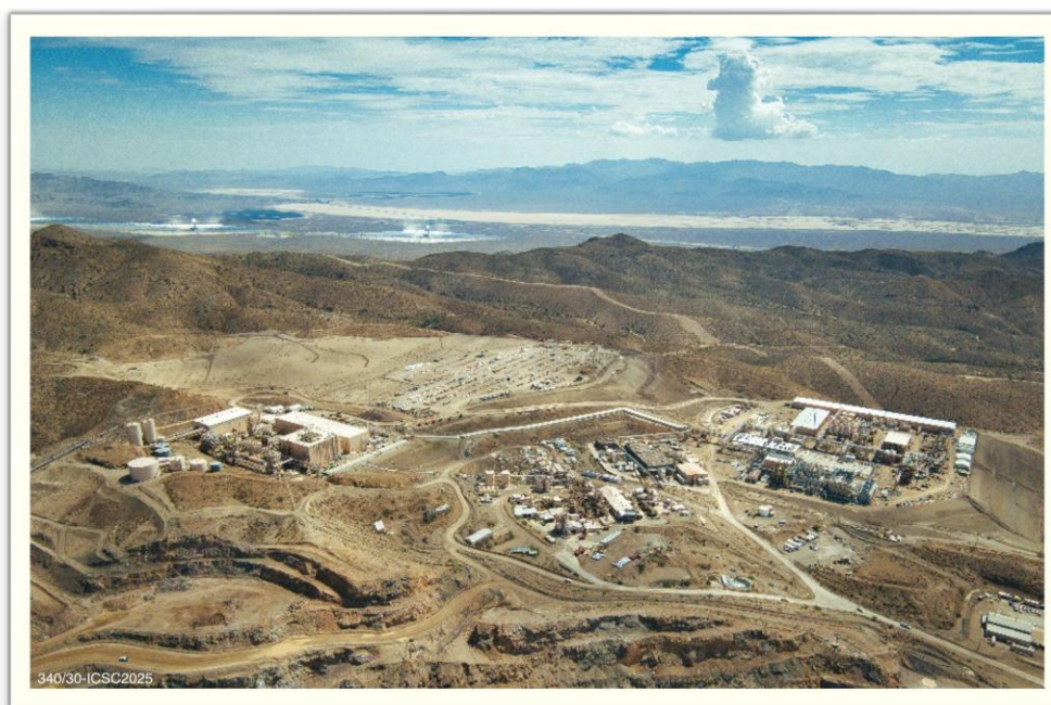
Figure 30 Mountain Pass rare earths mine in California, USA (courtesy of M P Materials)
