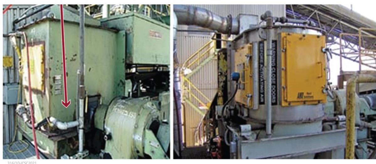
Figure 10 Fuel-handling equipment upgrade at Big Brown power plant, USA, to eliminate fuel build-up (Image courtesy of: Power)
