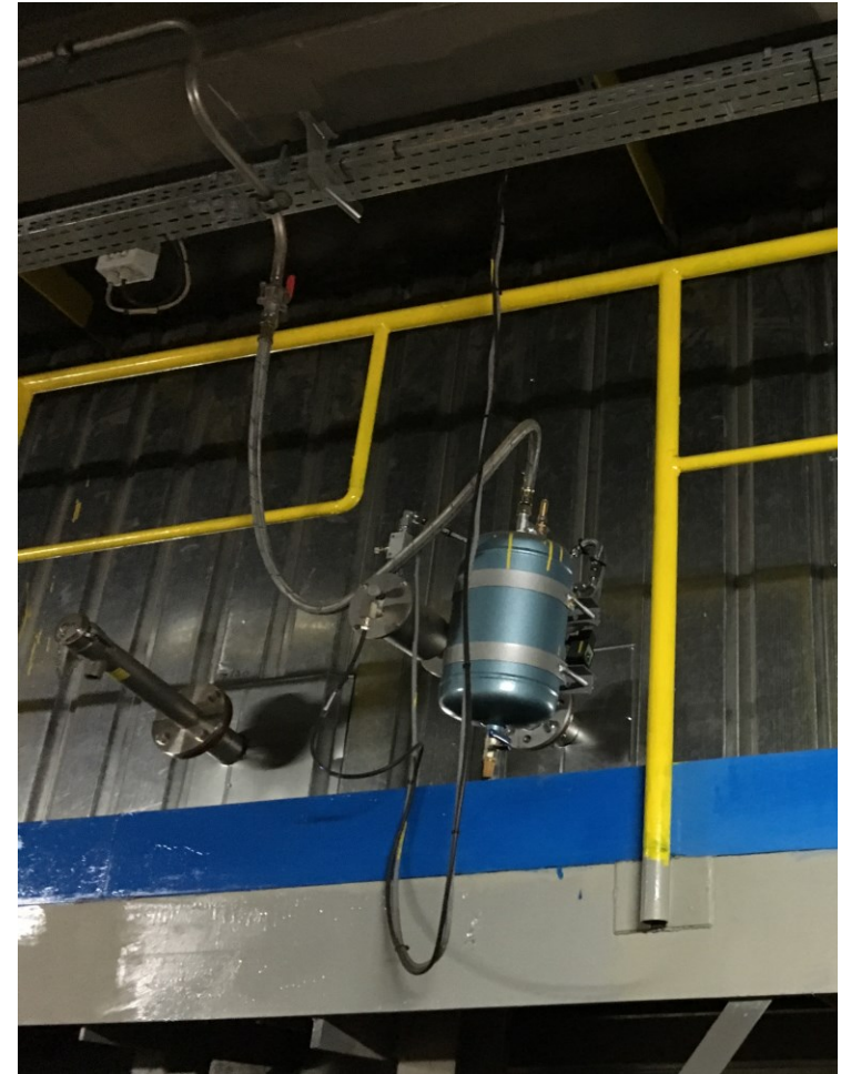
Pyrometer and Pyrometer with shock blower
