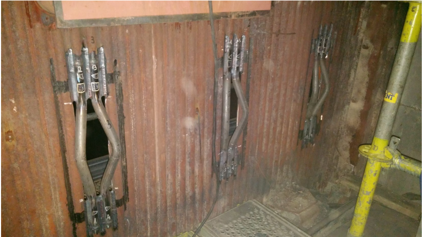
Openings in the Membrane Walls of the Furnaces
