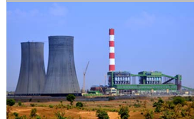
Maharashtra State Power Generation /Koradi SC 660MW x 3 25.0MPag/569/595°C
