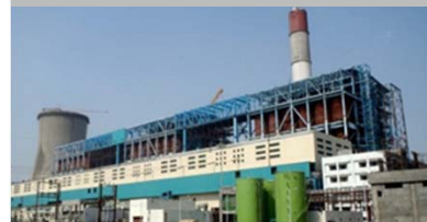
Maharashtra State Power Generation /Koradi SC 660MW x 3 25.0MPag/569/595°C
