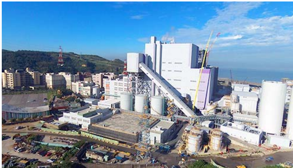
Taiwan Power Company's Linkou Thermal Power Plant
