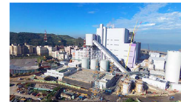
Taiwan Power Company's Linkou Thermal Power Plant
